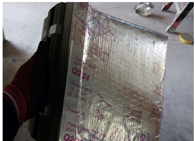
Fig. 2 The finished assembly. Fully wrapped and airtight before it goes up.
