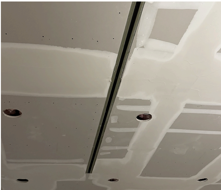
Fig. 5 Drywall hung around the diffuser, screwed off every 12 inches.
