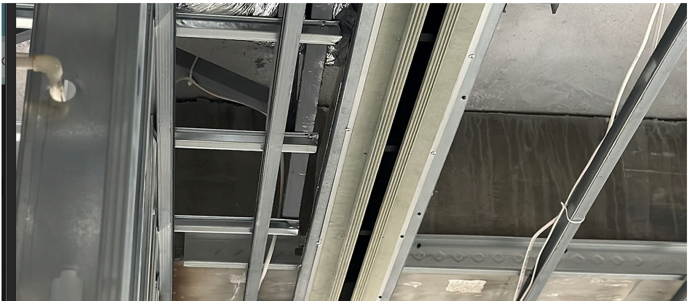
Fig. 3 The framed opening between joists. Straight and level here is what makes the drywall fit right three steps from now.
